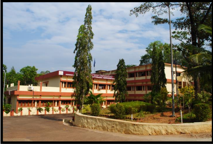
Figure 1 SCHOOL FRONT VIEW
