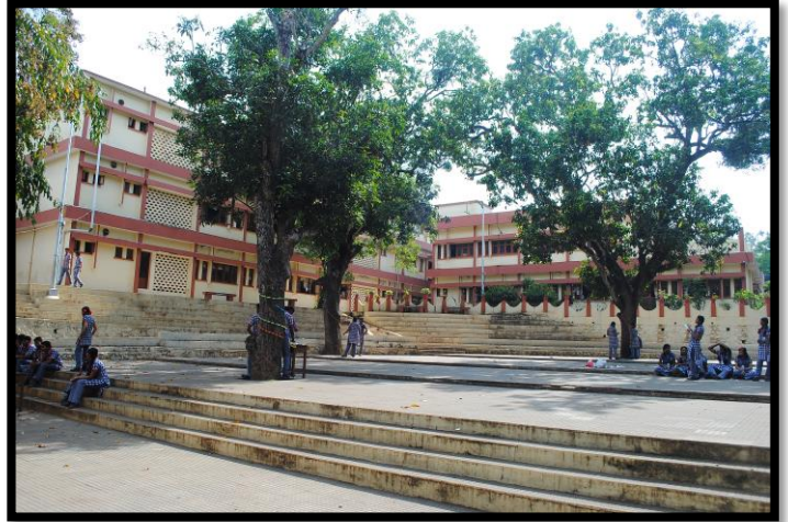
Figure 2 SCHOOL REAR VIEW
